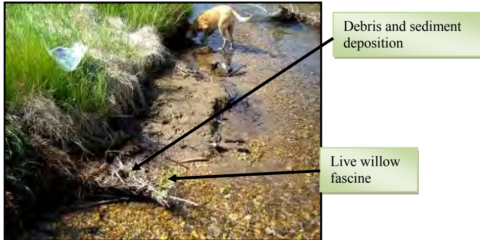
Figure 29. Photograph shows an example of sediment and debris deposition at the downstream end of a live willow fascine.
