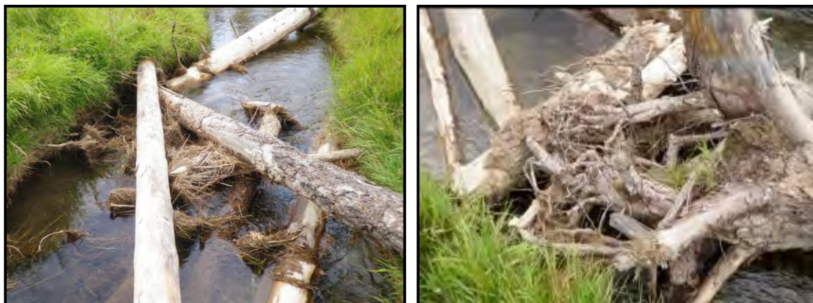
Figure 12. Photographs showing the accumulation of fine sediment and organic debris on large woody debris structure 1.
