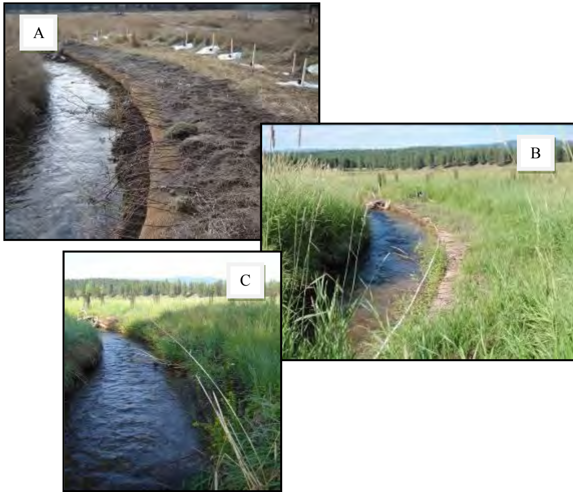
Figure 10. Photographs of Soil Lift 1 immediately after implementation (A), during July 2008 effectiveness monitoring (B), and during July 2009 effectiveness monitoring (C). Willow and herbaceous cover increased in 2009 on both the top and bottom layers of the lift.
